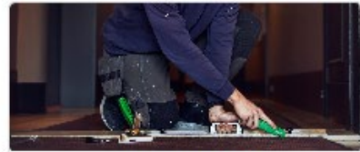
Modul 4 - Gulvlegging (Program)
